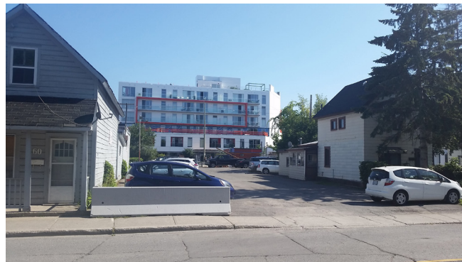
61 Armstrong Street looking towards Wellington West St
