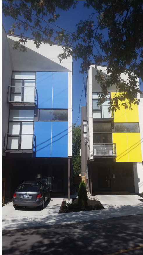
New residential buildings on Armstrong St
