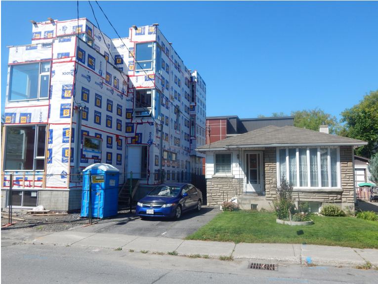
Apartment house in construction on Armstrong Street
