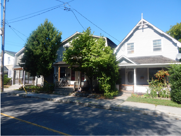
Residential houses on Armstrong Street
