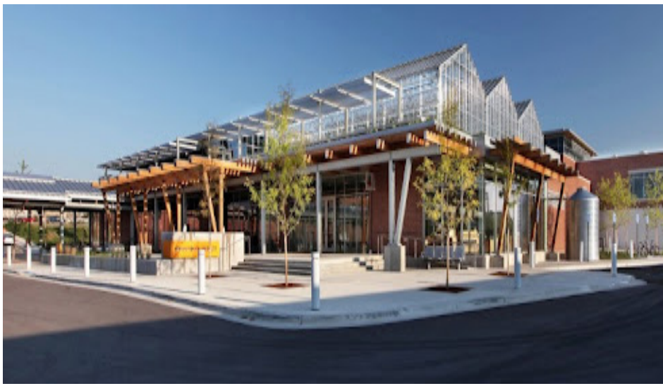
Figure 25: Grand Rapids Downtown Market building
