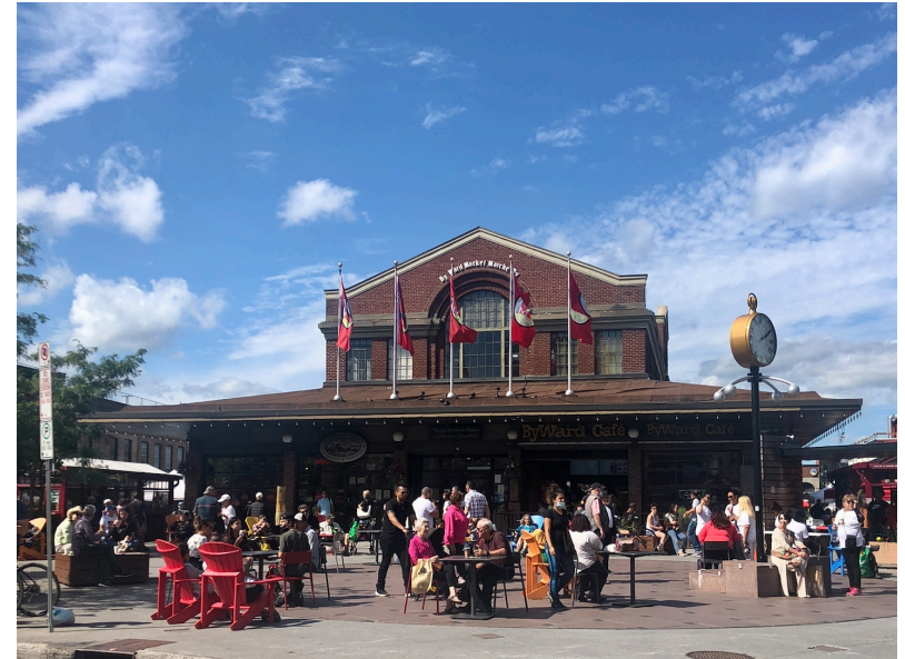
Figure 5: View of the exterior of the ByWard Market building from George Street
